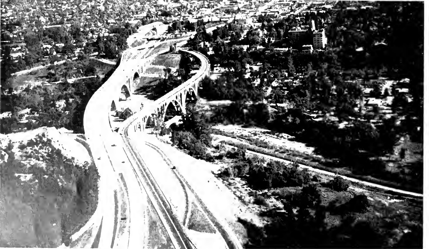
UPPER: Aerial view of highway interchange, Pasadena Freeway, showing Arroyo Seco storm drain channel foreground right, bridges crossing Los Angeles River in center. In background is area of Los Angeles River disposal area which state contractors, at considerable saving to the State, have hauled in some 5,000,000 cubic yards of excess excavated material in road's freeway project. In the foreground is shown area that will be traversed by future Golden State Freeway that crosses the Pasadena Freeway at approximately 90 degree angle. LOWER: Looking easterly along Colorado Freeway showing Pasadena Pioneer's Bridge over Arroyo Seco on left and Old Calaveras Street Bridge on right with Pasadena Civic Center and business district in background.
